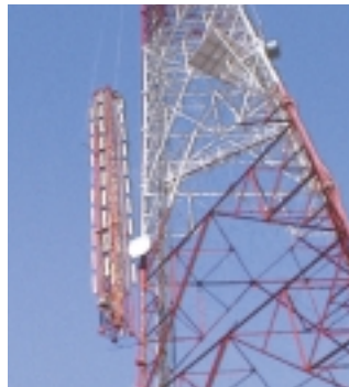
WUSA-TV's new digital/UHF antenna is hoisted to the top of the tower.
